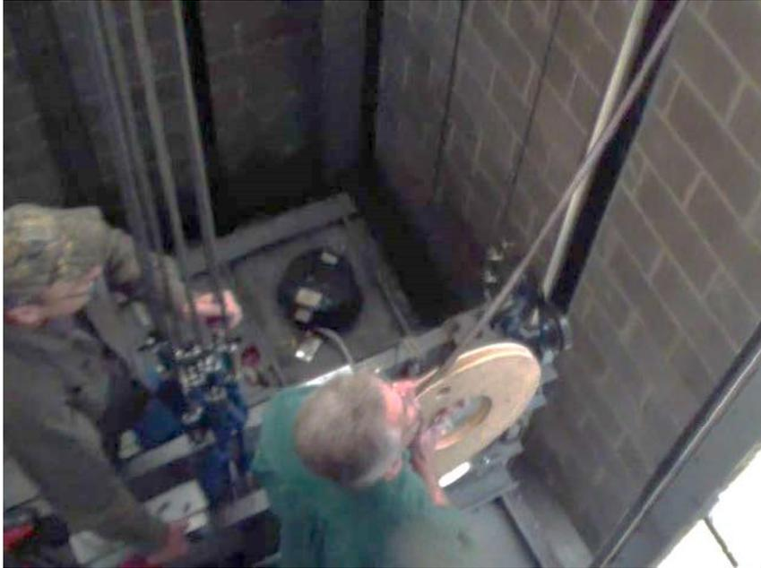
Figure 2-5: Unroll the Encoded Tape
