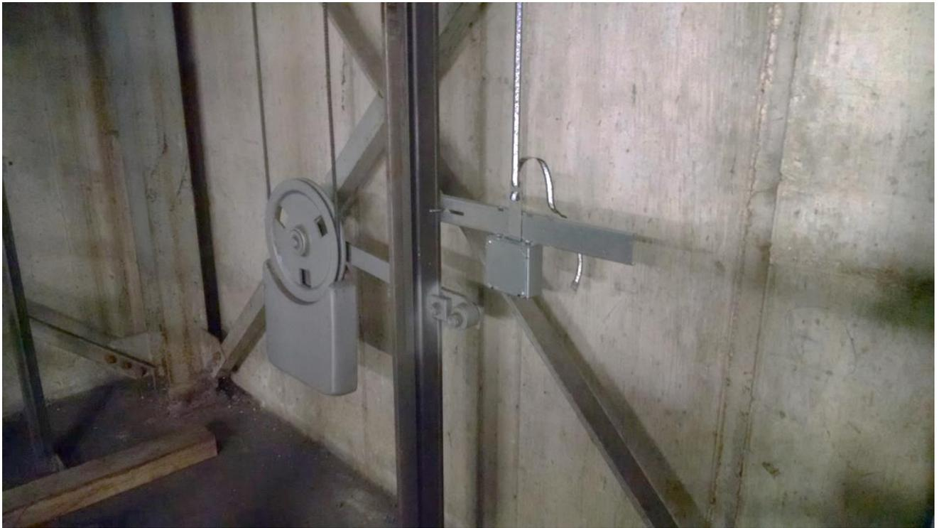
**Figure 2-8: Encoded Tape Mounting – Bottom Bracket**
