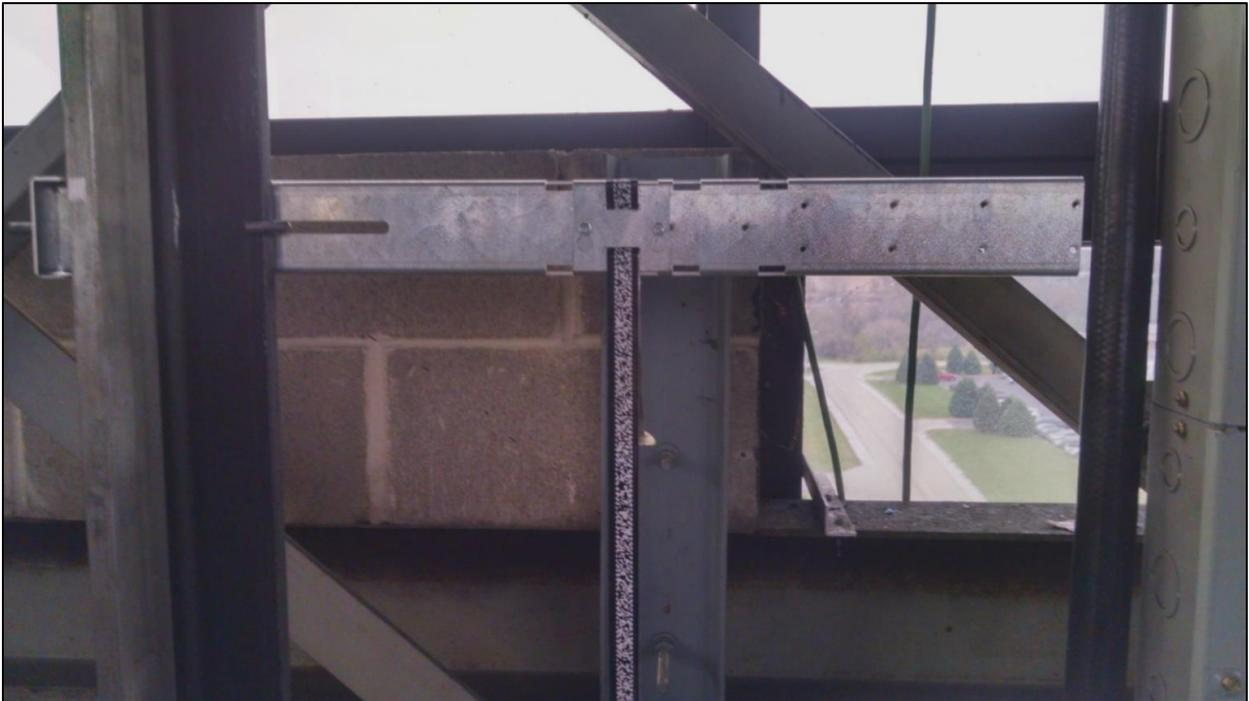
**Figure 2-2: Encoded Tape Mounting – Top Bracket**
